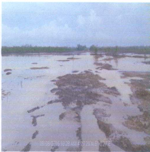
Fig D: picture taken after backfilled.
