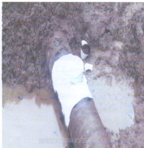
Fig C: picture taken after wrapped.
