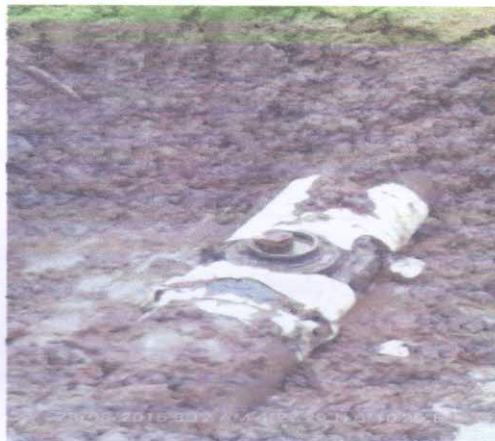
Fig B: picture taken after excavation.
